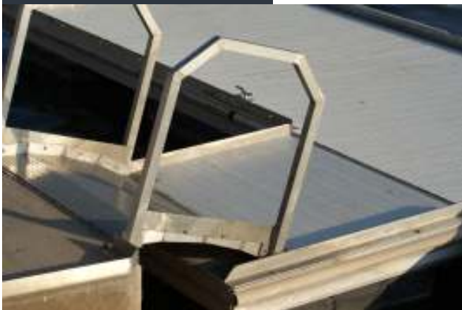
Soon to be completed, Tempe strives to make Town Lake Accessible for All
